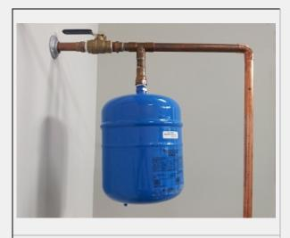
Install a thermal expansion tank to protect your plumbing system and water heater.
